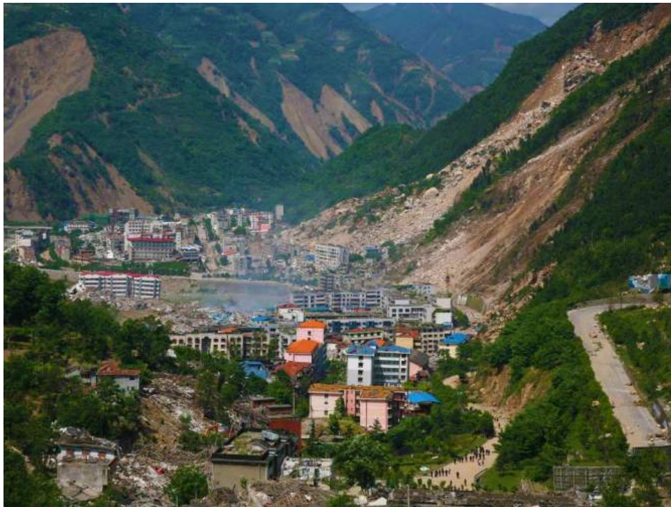
Fig. 4 Disaster in Beichuan town where landslides triggered by the Wenchuan Ms 8.0 earthquake caused thousands of deaths (T2)
