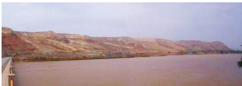
Fig. 3 The Heifangtai loess landslide cluster of Yongjin County, Gansu Province (T1)
