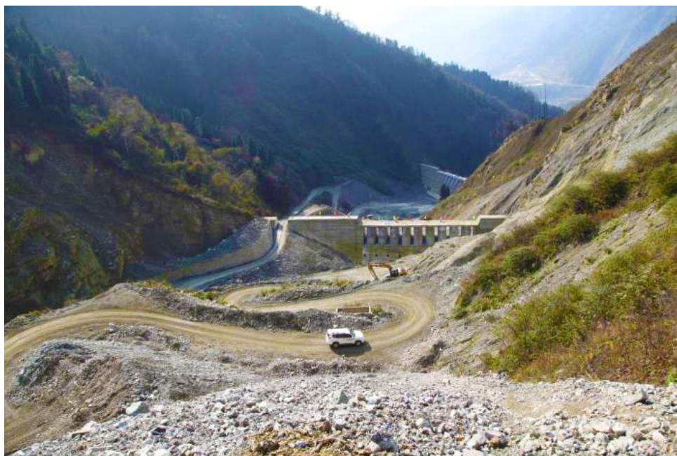
Fig. 5 Prevention measures undertaken in 2012 to reduce the debris flows hazard after the 2008 Wenchuan Earthquake (T2).
