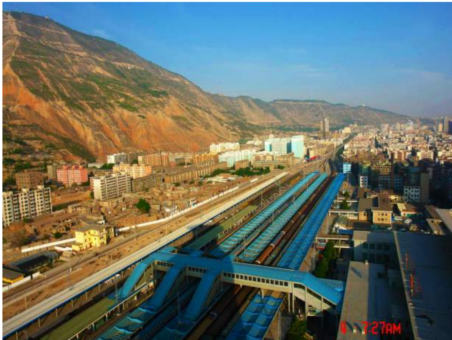
Fig. 2 The 20.56 million m 3 Gaolanshan landslide located on the southern side of Lanzhou City (T1) It consists of three sub-landslides, with multiple layers and multiple activities. The slope height is about 600 m and landslides endanger the district below it.
